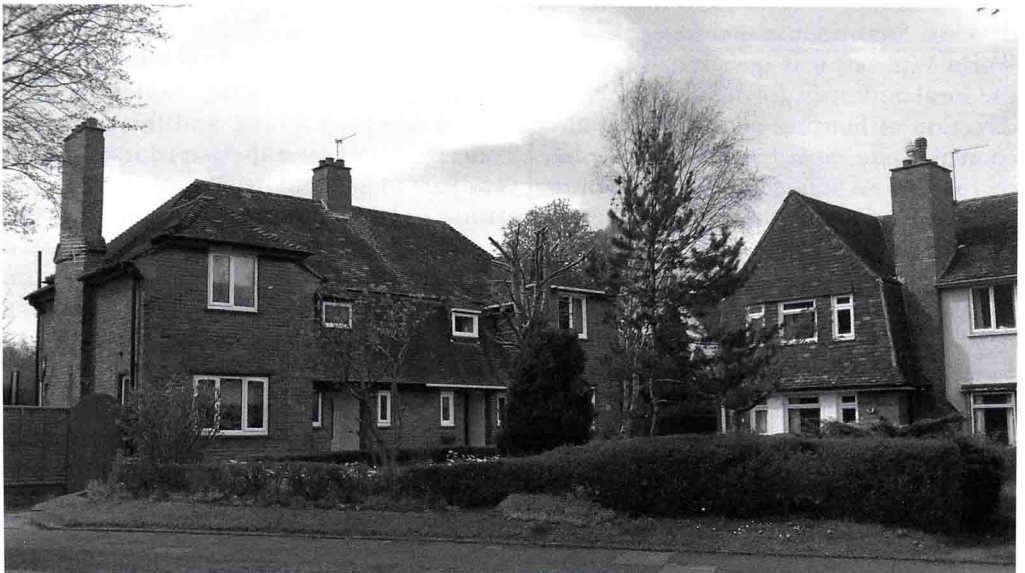
2 Early council housing, Chaucer Drive, St Giles estate, Lincoln
